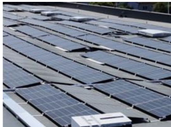
Figure 2: East-west PV module orientation
